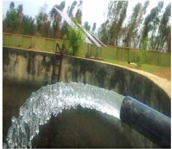
5 HP AC Submersible Solar Pump installed at Alamathy, Chennai
