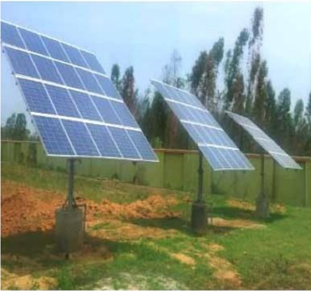
5 HP AC Submersible Solar Pump installed at Alamathy, Chennai
